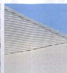
SR1 SURFMIST METAL DECK ROOF
